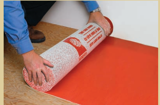
1. Install foam underlayment
