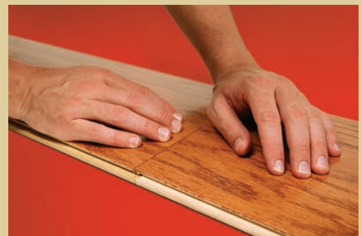
2. Engage long sides at an angle
