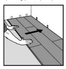
10. Last row (and perhaps also first row). Minimum width must be at least 2" (50mm). Remember to leave an expansion gap of 3/8" (10mm).
