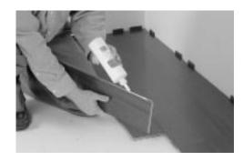
ArborCraft Floating Wood Floors can be installed above grade, on grade, or below grade. When installing over concrete or below grade a moisture barrier of 6-8 mil plastic sheeting is required. Loose lay the sheeting with the seams overlapped 8 inches, and lapped up the wall 4 inches. The plastic can be trimmed at the walls after the molding is installed.
